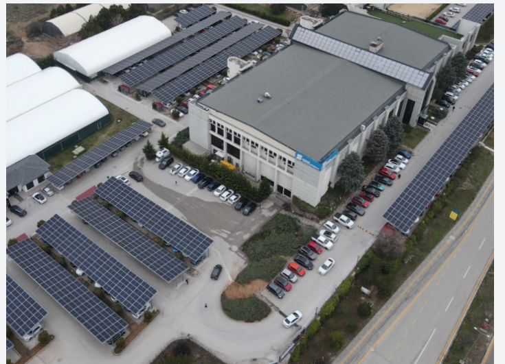
Bilkent Sports Carport GES, 0.8 MW, Ankara
