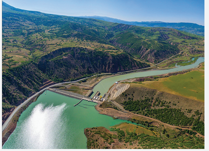
Özaltın Holding, Yedisu HES, 21 MW, Bingöl
