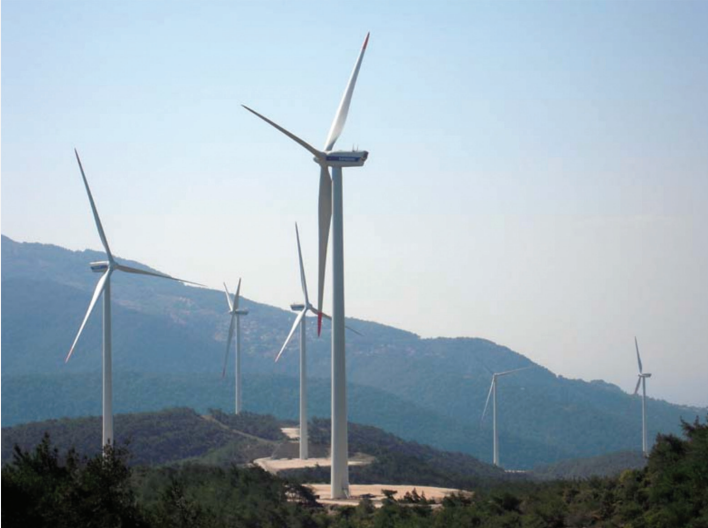
Akfen Holding, Belen RES, 35 MW, Hatay
