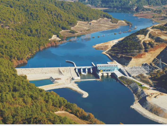
Enova Enerji, Ceyhan HES, 65 MW, Osmaniye
